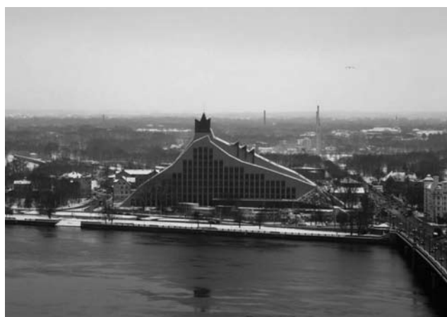
Image 2. The new building of the NLL in December 2012
