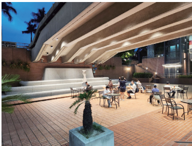
戶外休憩區照明優化 Improved lighting for the outdoor space.
