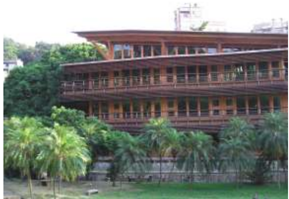
Exterior view of the Taipei Public Library's new Beitou branch
